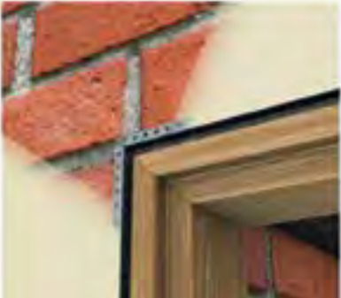
DOOR JAMB WITH SHADOW EFFECT USING R50
