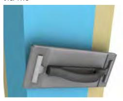
Using sandpaper and sanding float, gently sand the dry joints to a smooth even finish. Hold the float diagonally across the joint, taking care not to scuff the paper face of the building board where it meets the setting compound.
