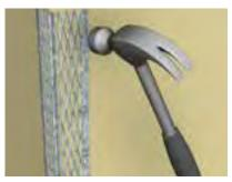
Beads can be attached by nails or a staple gun at not more than 500mm centres down the legs of the bead, and not more than 4" from each end.
