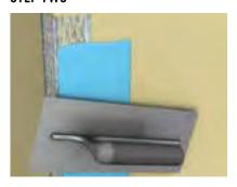
Using a 4"broad knife, apply setting compound to the bead to a width of approximately 4"each side of the corner, filling all perforations.
