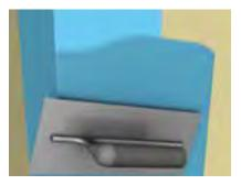
Apply third coat with a 8" broad knife. Feather edges with a wet paint brush. Allow to dry.
